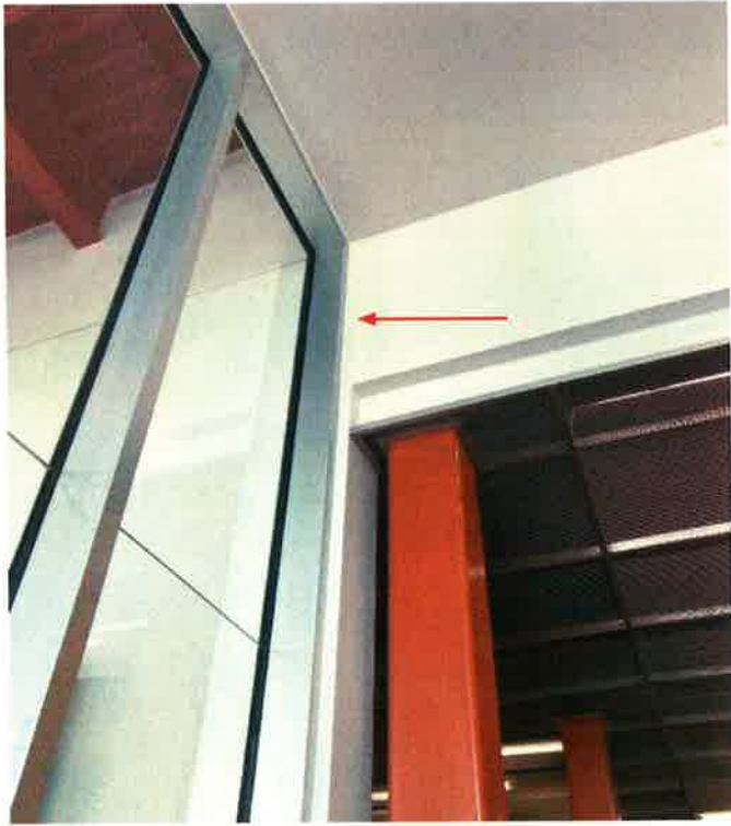
#7. Gypsum board wall cracks
