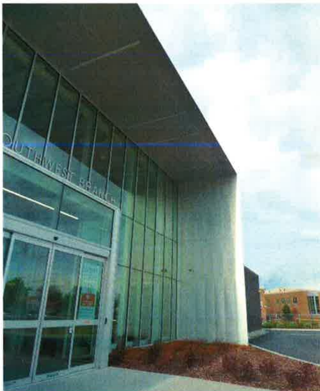
No apparent damage was observed at North entrance
