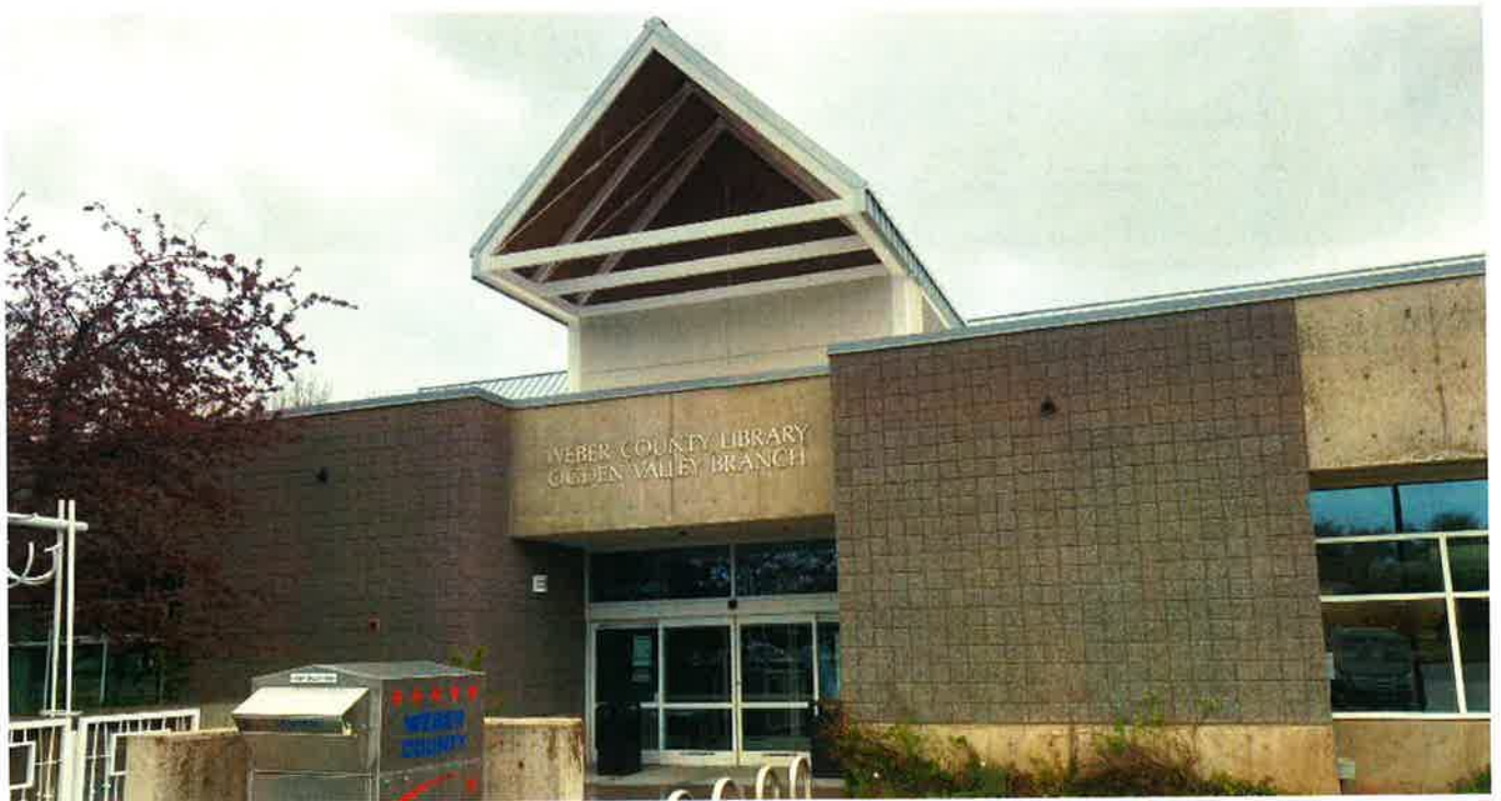
No damage was exhibited at the Main entrance
