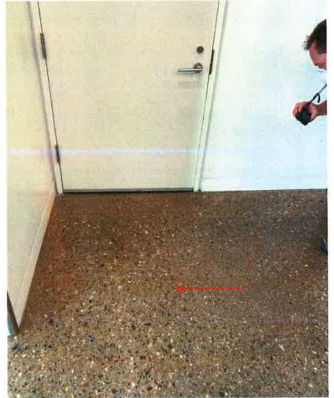
#6. Concrete floor cracks
