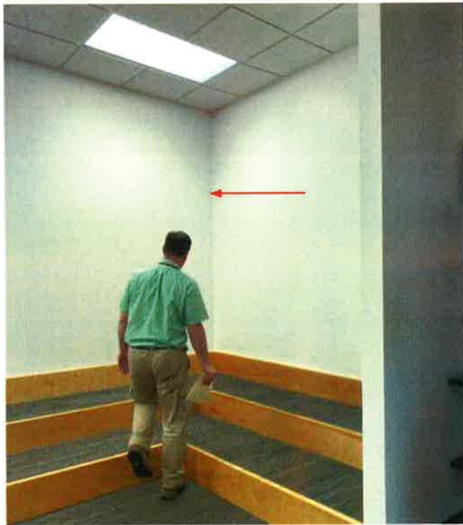
#6. The Children's Area exhibited gypsum board wall cracking
