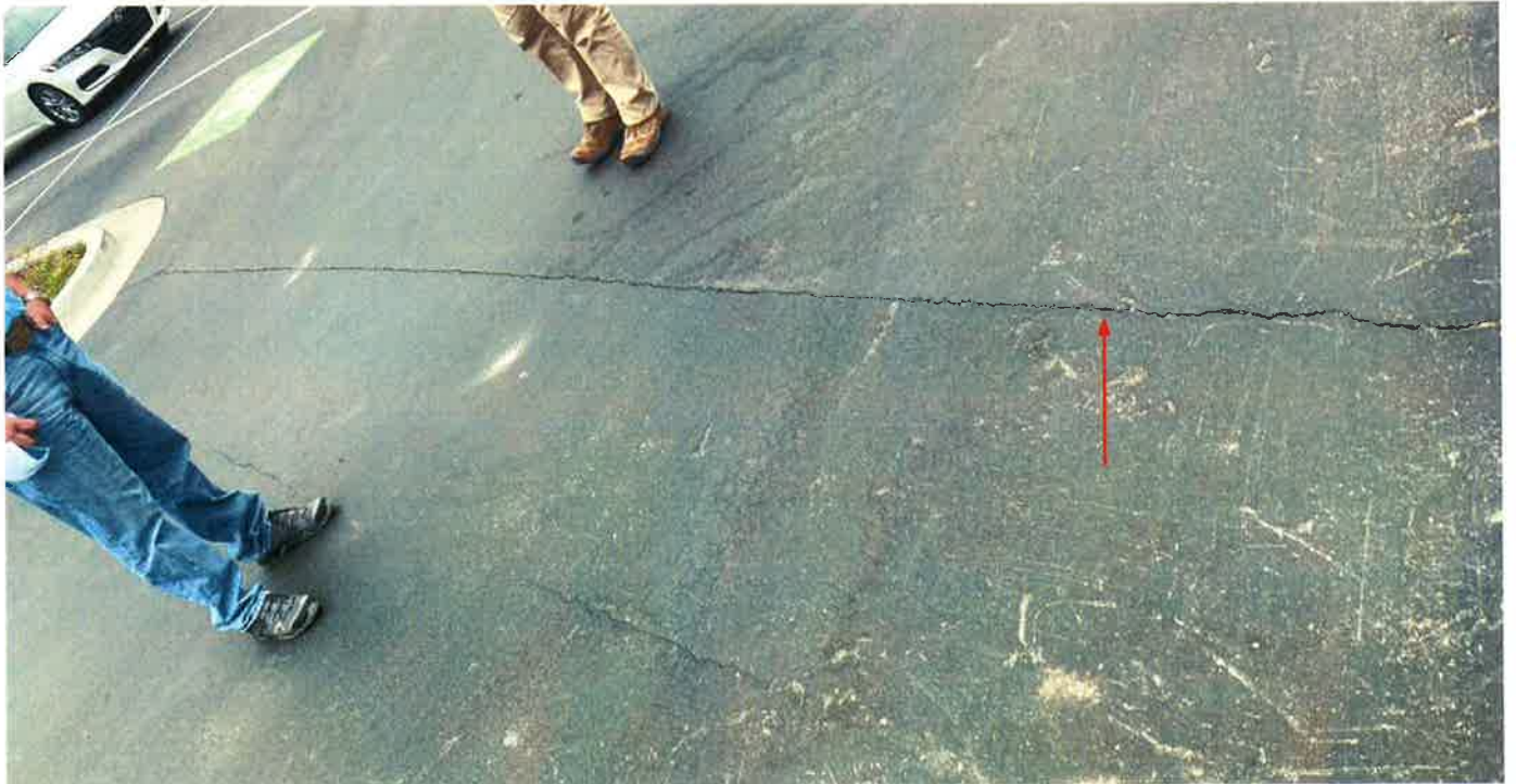
# 1. Asphalt surface crack at parking lot
