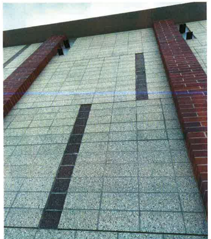
Brick and CMU does not show sign of damage
