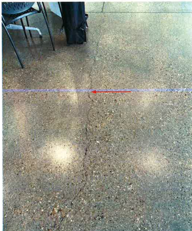
#6. Concrete floor cracks at public circulation areas
