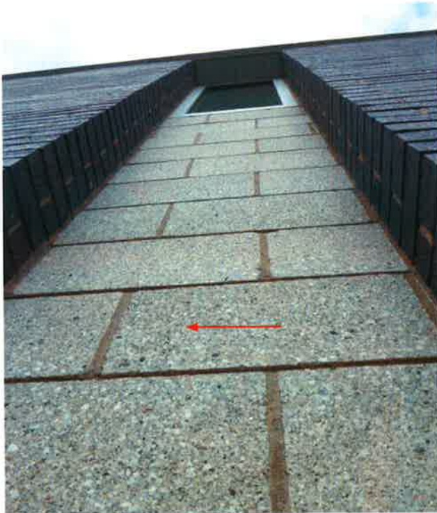
#2. Hairline cracking at CMU Walls: North and West Facades
