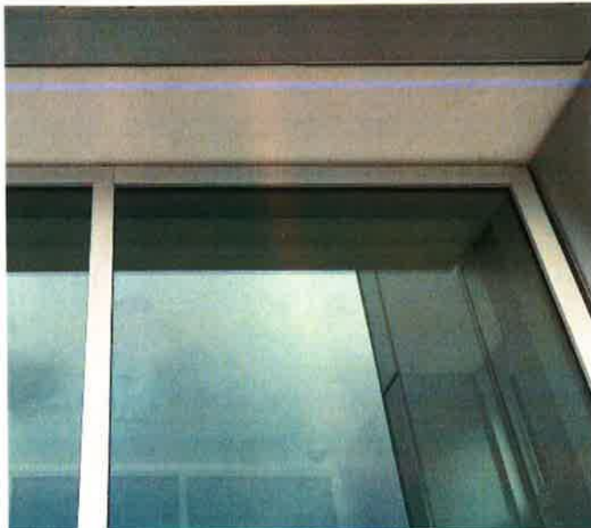
#2. Lower level South entrance glazing
