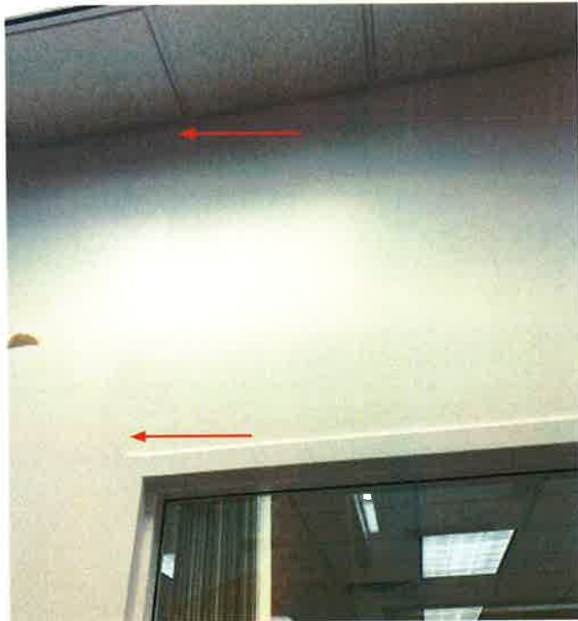
#3. Hairline cracking near door frames
