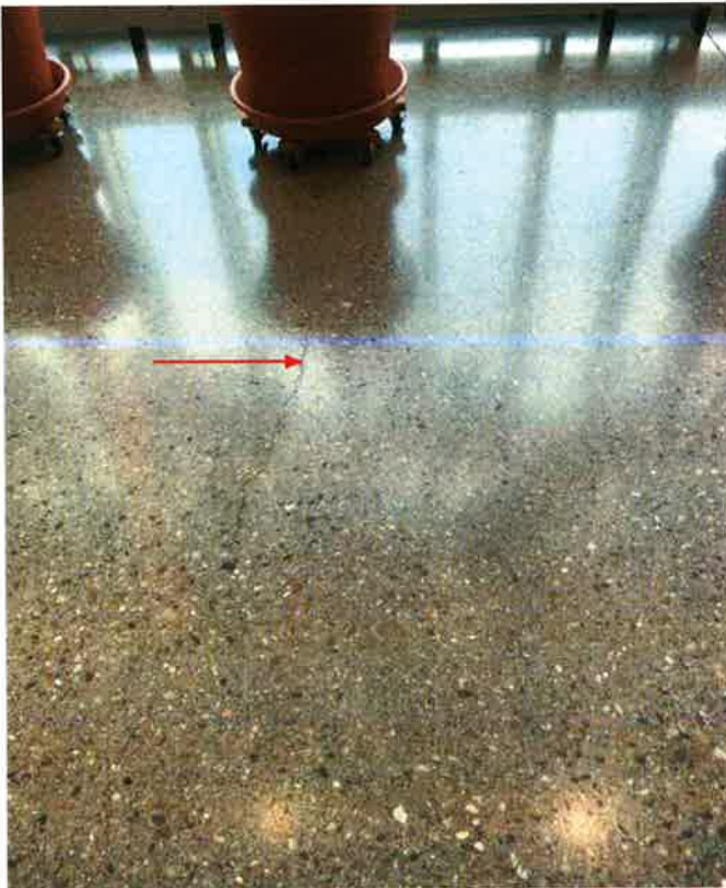
#6. Concrete floor cracks at public circulation areas
