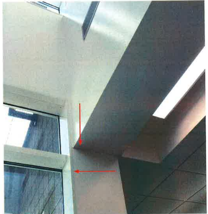
#3. Hairline crack at painted gypsum wall surface
