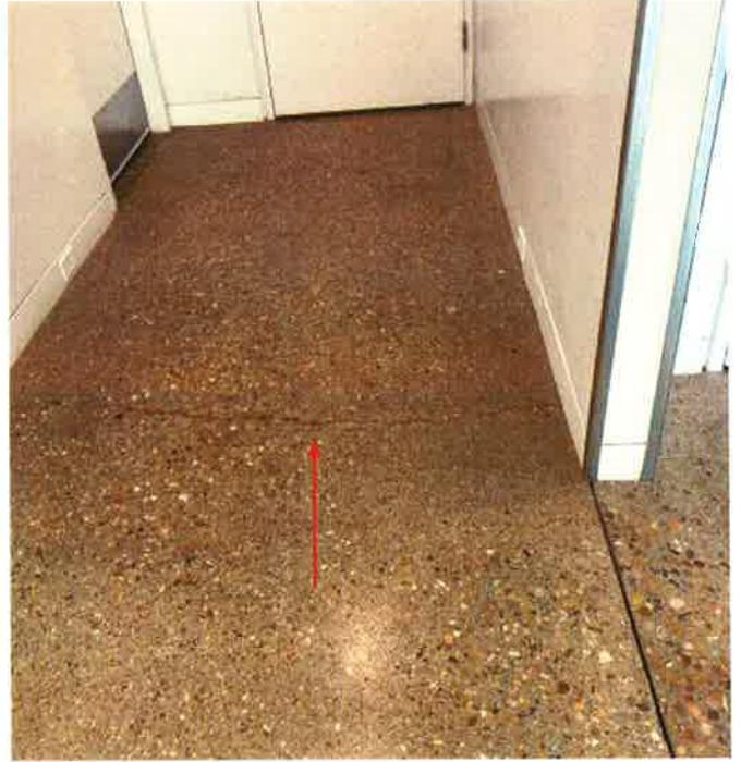
#6. Concrete floor cracks
