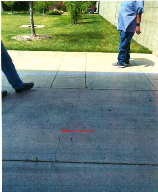
#2. Cracks at entrance walkway concrete slab on grade
