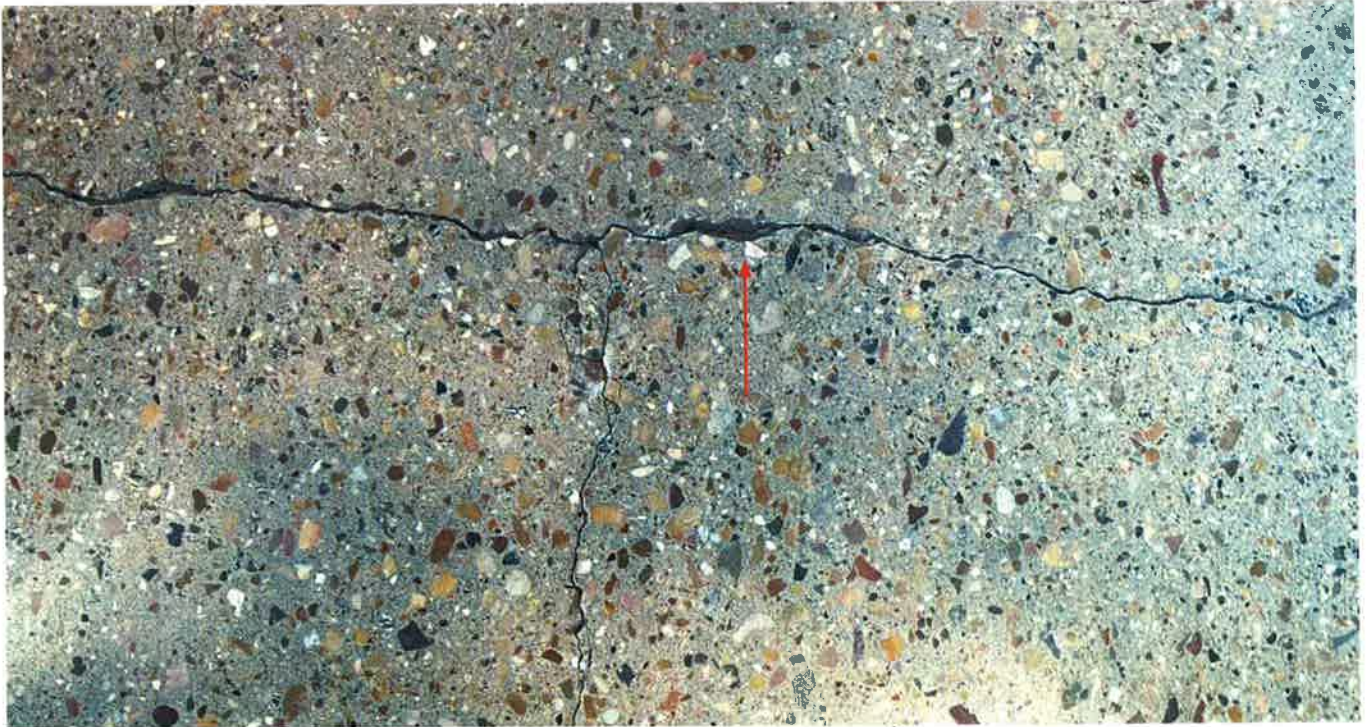
#6. Concrete floor cracks at public circulation areas
